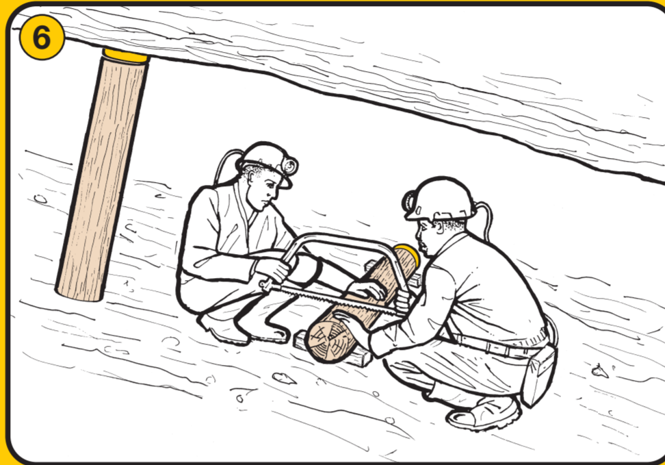
6. Cut the pole exactly to your measurement. A straight cut will reduce the amount of pumping required. Do not cut the end which holds the Jackpot, always cut the free end of the pole.
