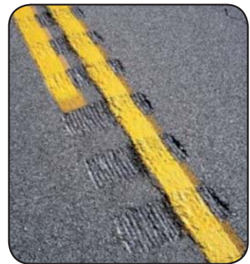
Figure 2. Rumble strips
