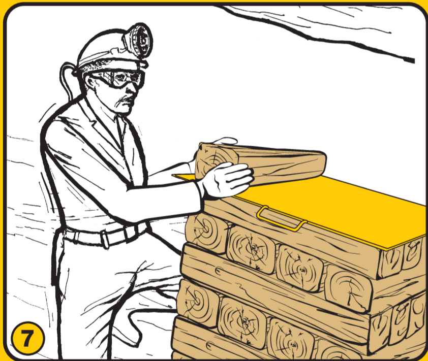
7. Build the rest of the timber pack up to the hanging-wall. Make sure the pack fits tightly to reduce the amount of pumping needed.
