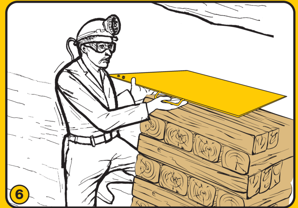
6. Place the Jackpack onto the timber pack before the pack reaches the hanging-wall. Make sure that the valve is facing away from the blasting direction.
